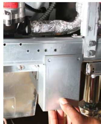
Figure 13: Position the thermostat protective cover over the thermostat and mount with drill-point screws.
