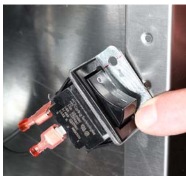
Figure 9: Switch being positioned on JIB cabinet right interior (front view).
