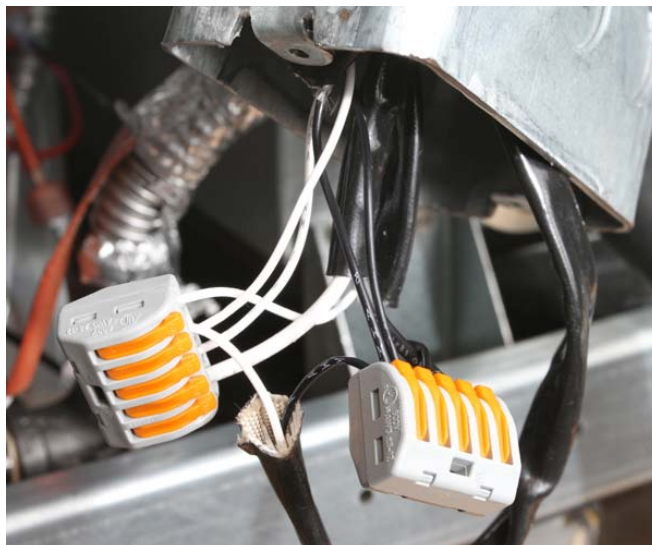
Figure 28: Wago connectors shown in junction box.
