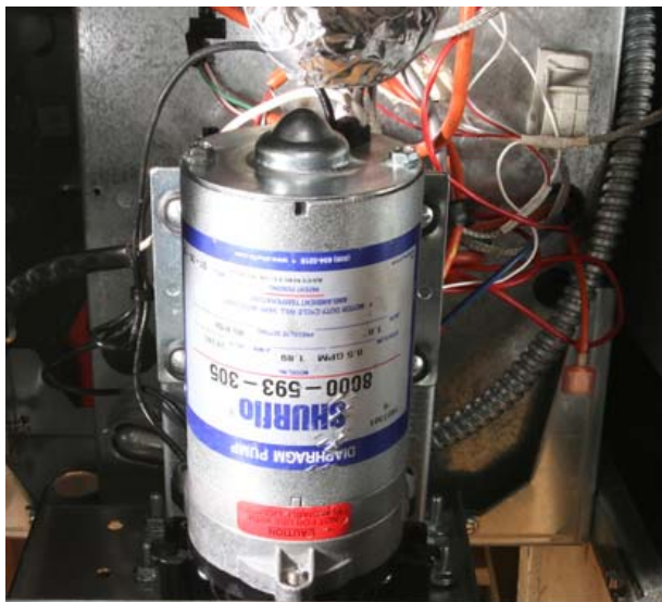
Figure 6: Position the pump on the provided bracket.
