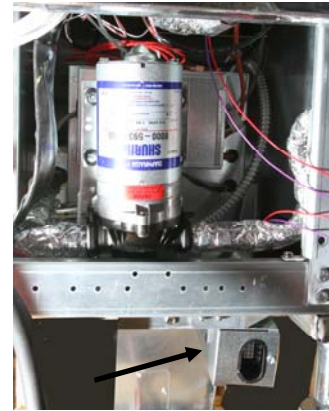
Figure 11: Mount the thermostat housing under the ATO pump bracket.
